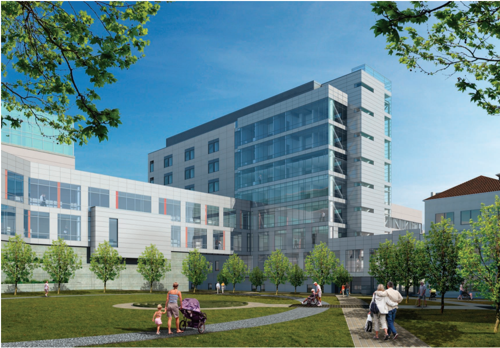
The Highland Hospital Acute Tower Replacement Project - Alameda County's largest capital project, scheduled for completion in 2017.
